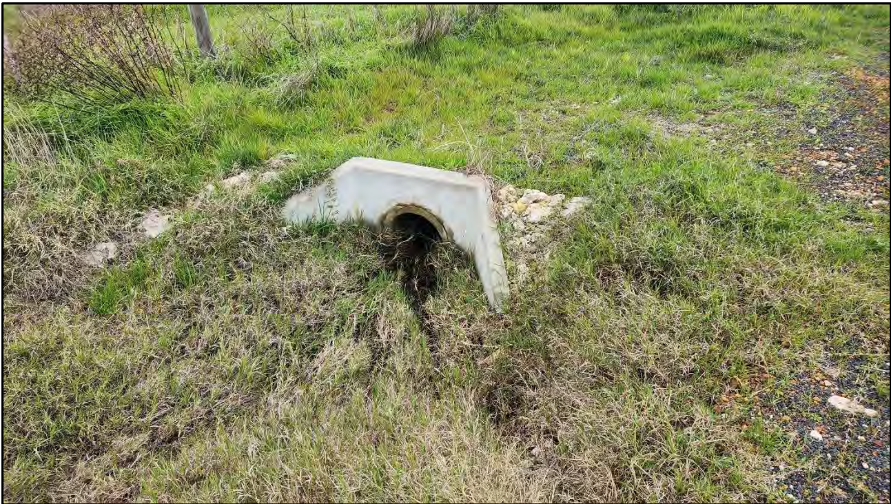
Photo 1: DN300 culvert within Ayrshire Rd discharging runoff into basin within catchment E4.
