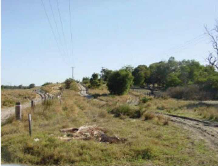
Figure 15 22 kV line along Temple Road Reserve
