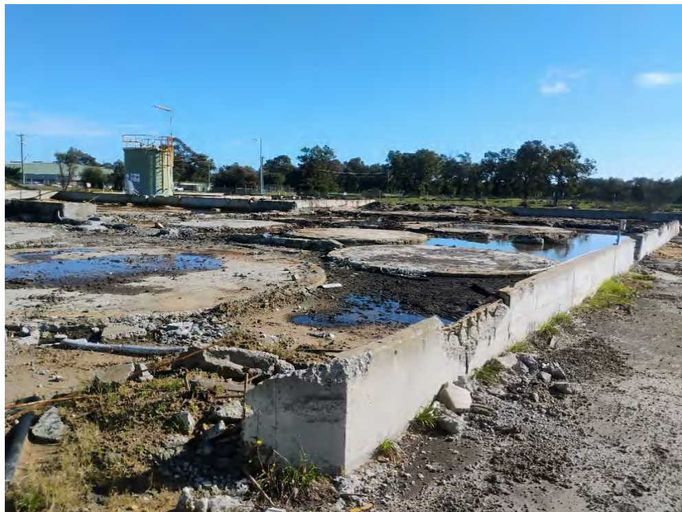
Photo 4: Former bio-diesel storage tanks
