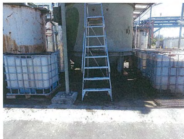
Photograph 3 – Waste oil sump
