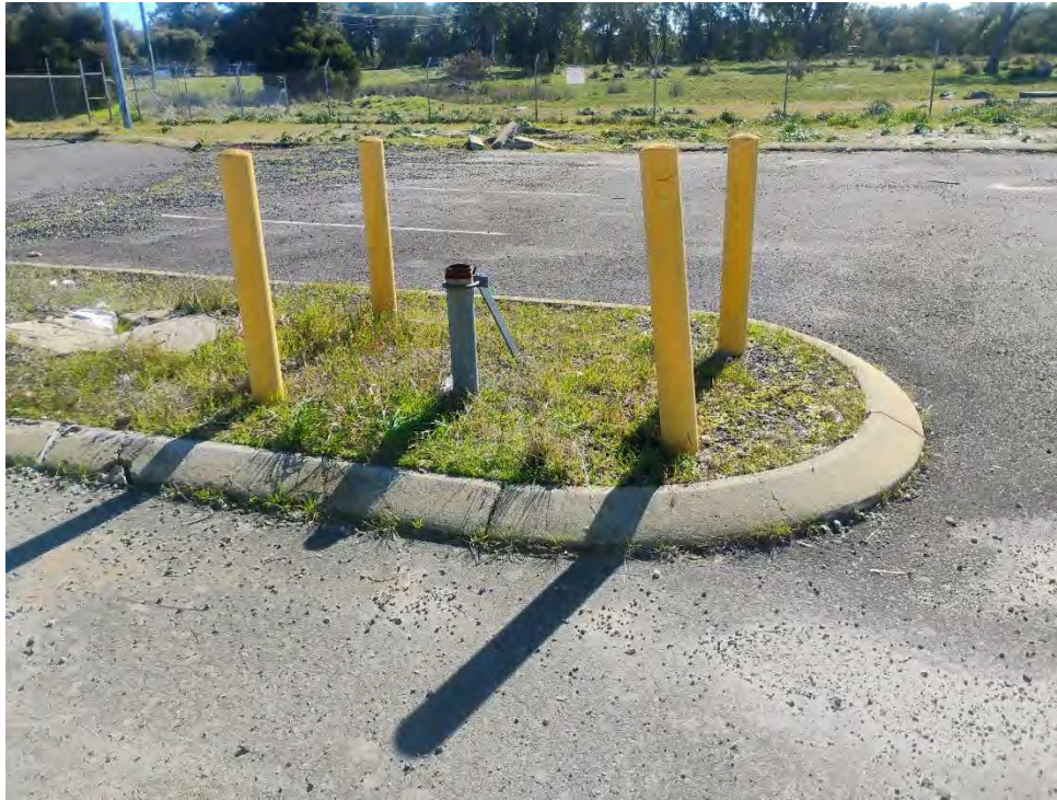
Photo 11: Metal riser (possible groundwater monitoring well)
