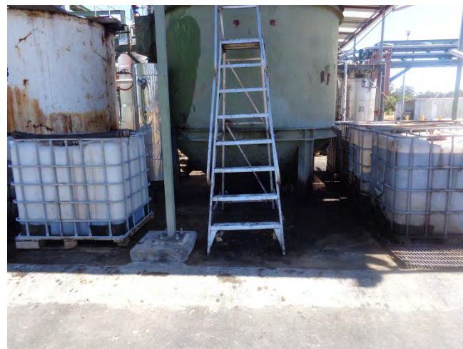
Photograph 3 – Waste oil sump
