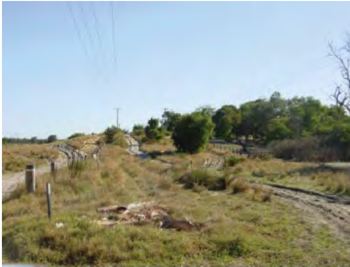
Figure 15 22 kV line along Temple Road Reserve
