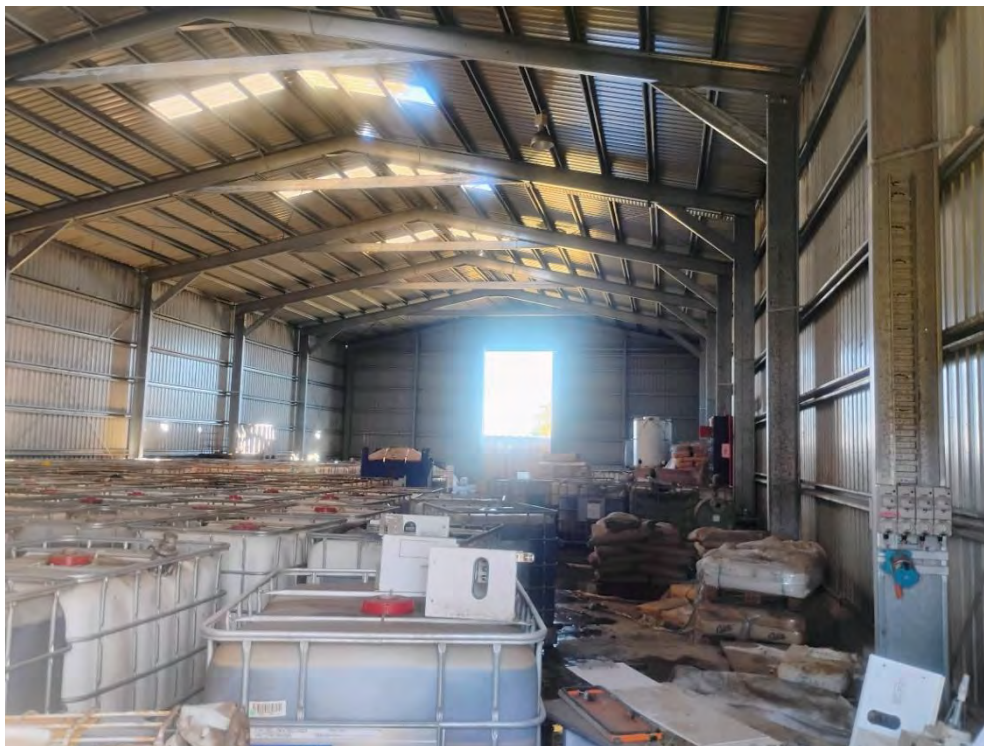
Photo 5: Inside storage shed with IBCs
