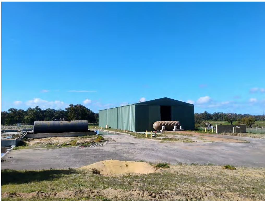
Photo 1: Looking towards the metal shed and tanks in the southwestern portion of the site
