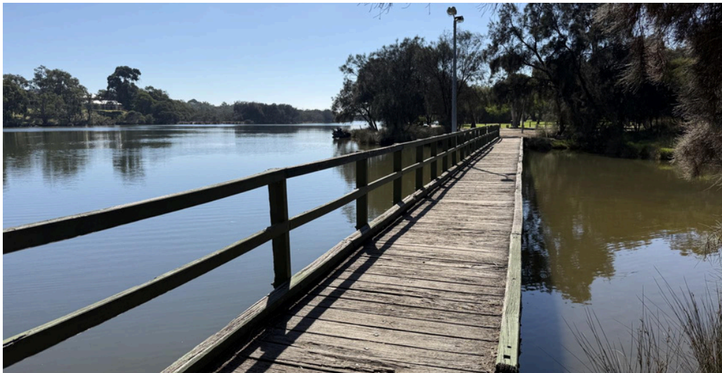
The Watsons Reserve footbridge is temporarily closed for about six weeks while it is being replaced.
