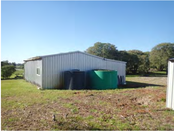
Photo location 26: existing water tanks and sheds within the site, looking north-east.
