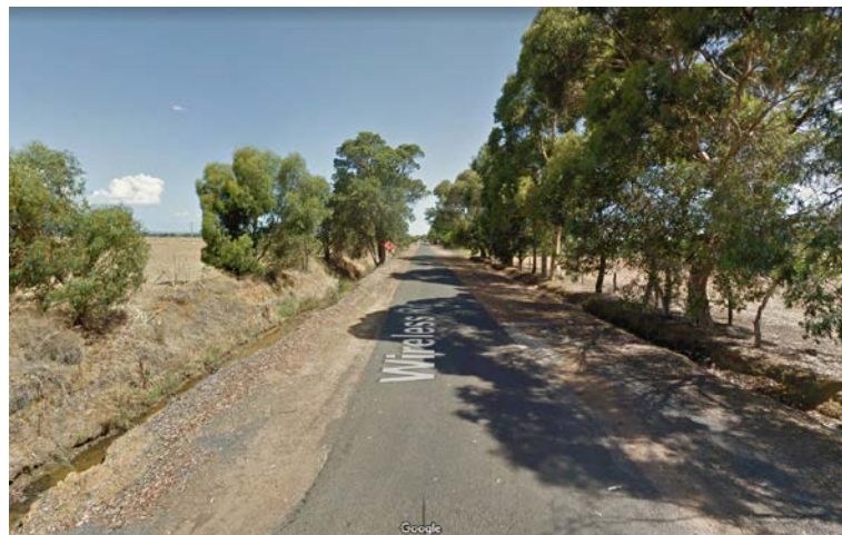
Existing Wireless Road - will remain after the BORR is completed
