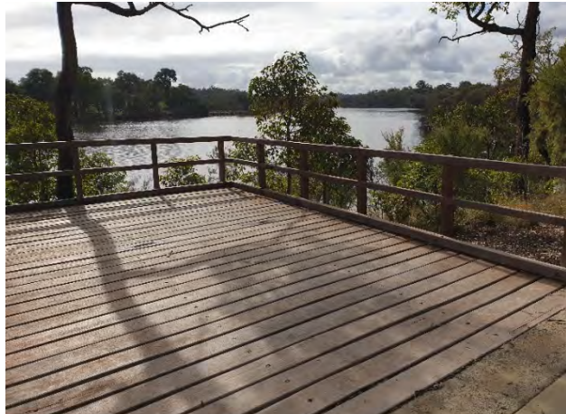
Lookout overlooking Collie River in the Shire of Dardanup's Pratt Road Reserve. Photo – Paul Roberts/DBCA
