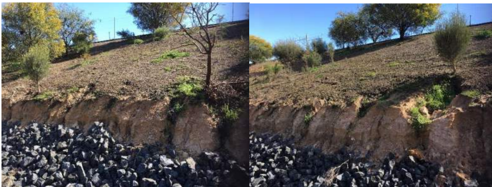
Images 1 & 2. Southern boundary bund, September 2021.
