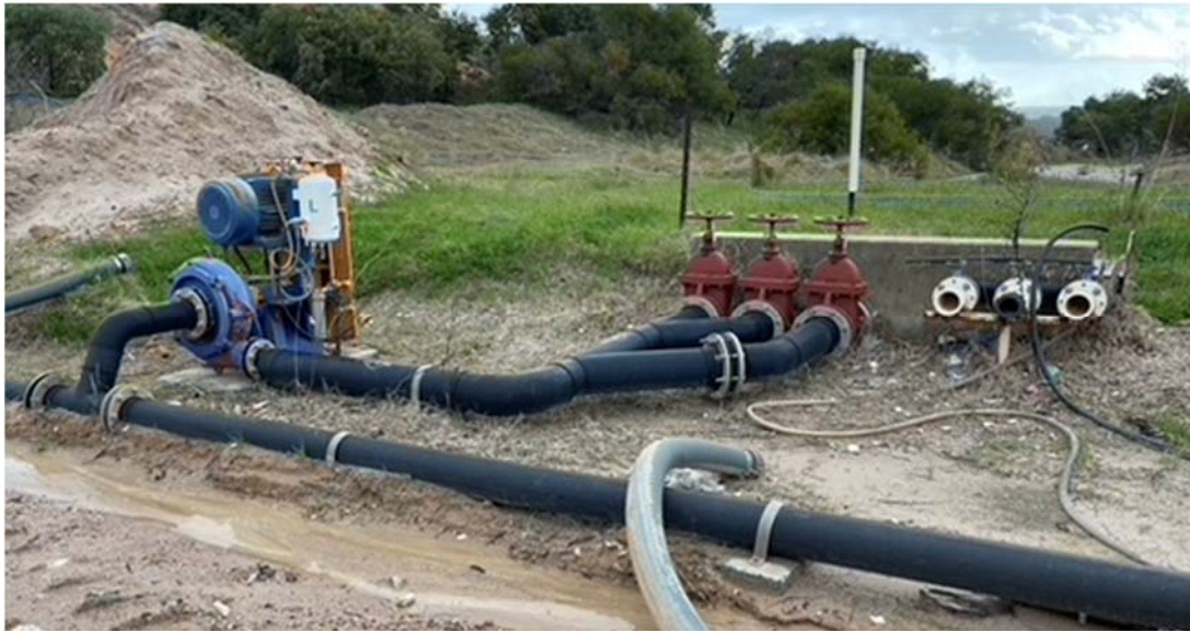
Figure 6 – Existing tailings disposal point
