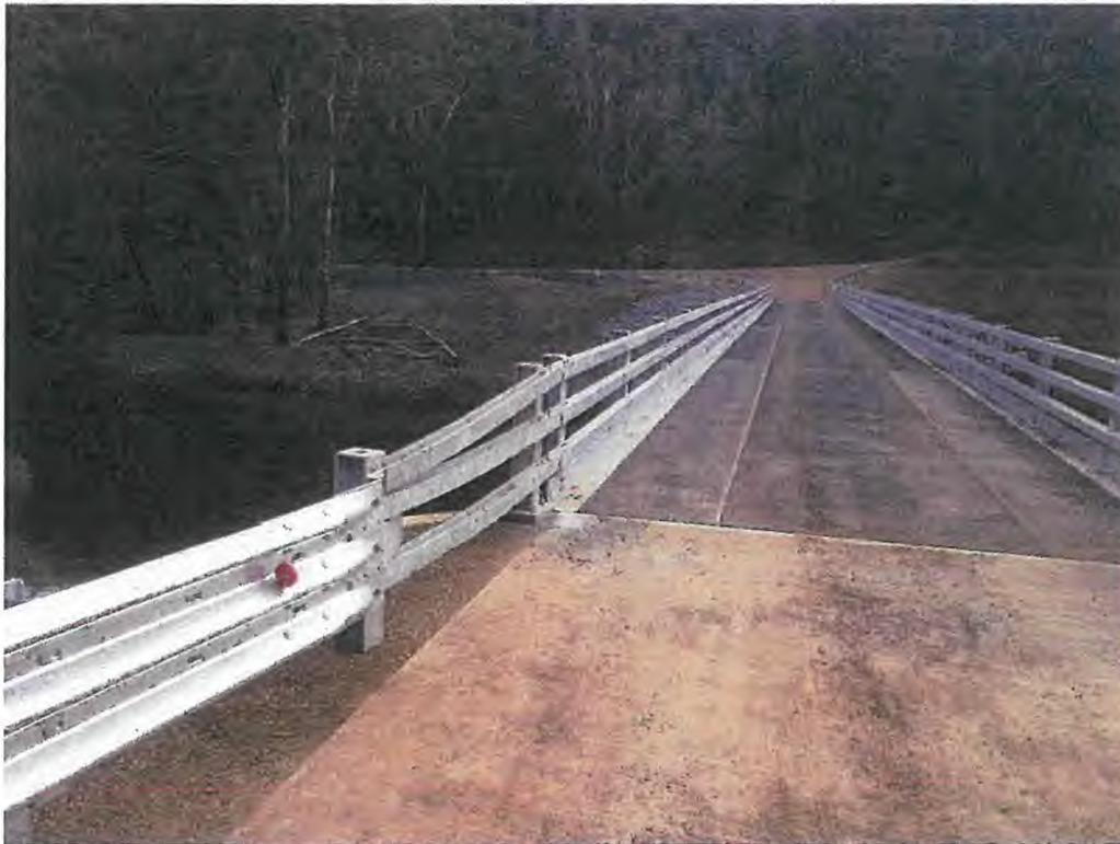
Photo No. 1: Abut 1 LHS (Taken: 25-Jun-2015)
