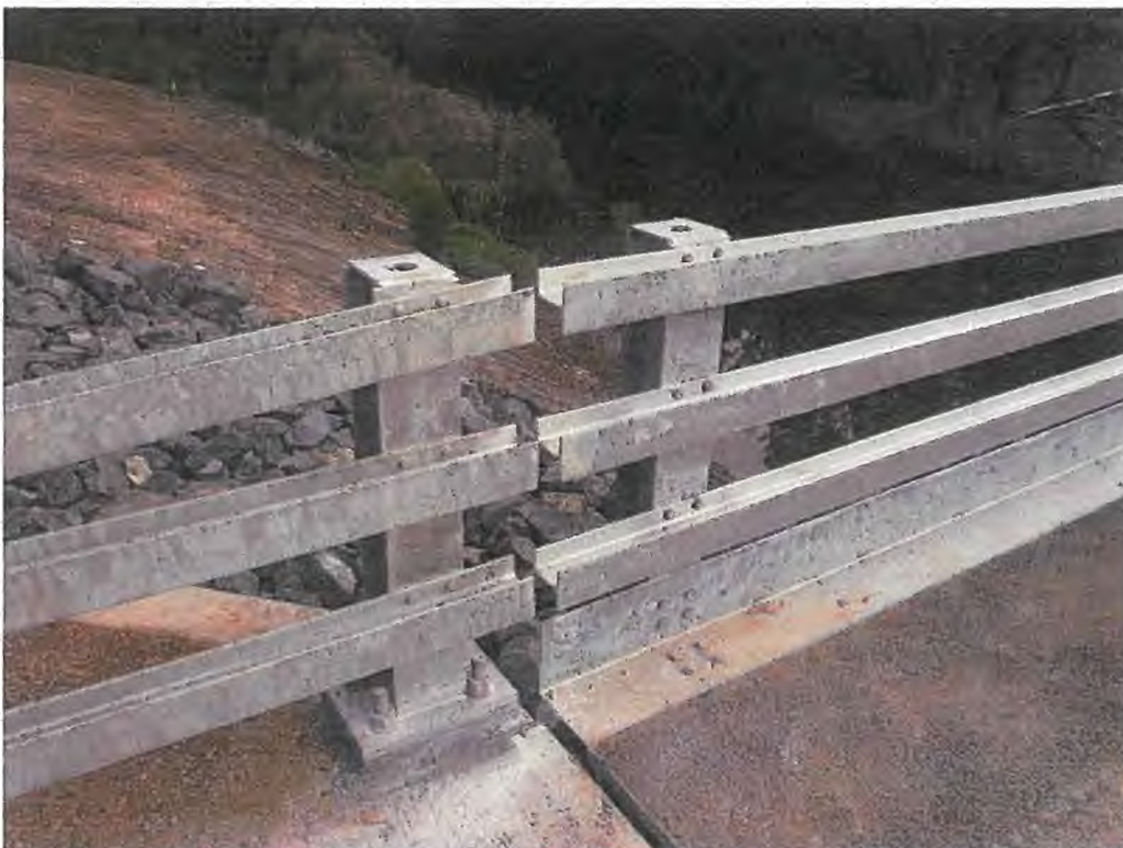
Photo No. 2: Abut 1 LHS guardrail transition (Taken: 25-Jun-2015)
