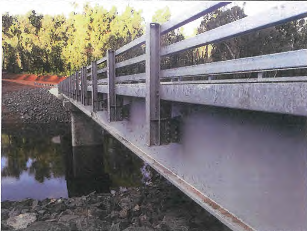
Photo No. 1: RHS viewed from Abut 2 (Taken: 25-Jun-2015)
