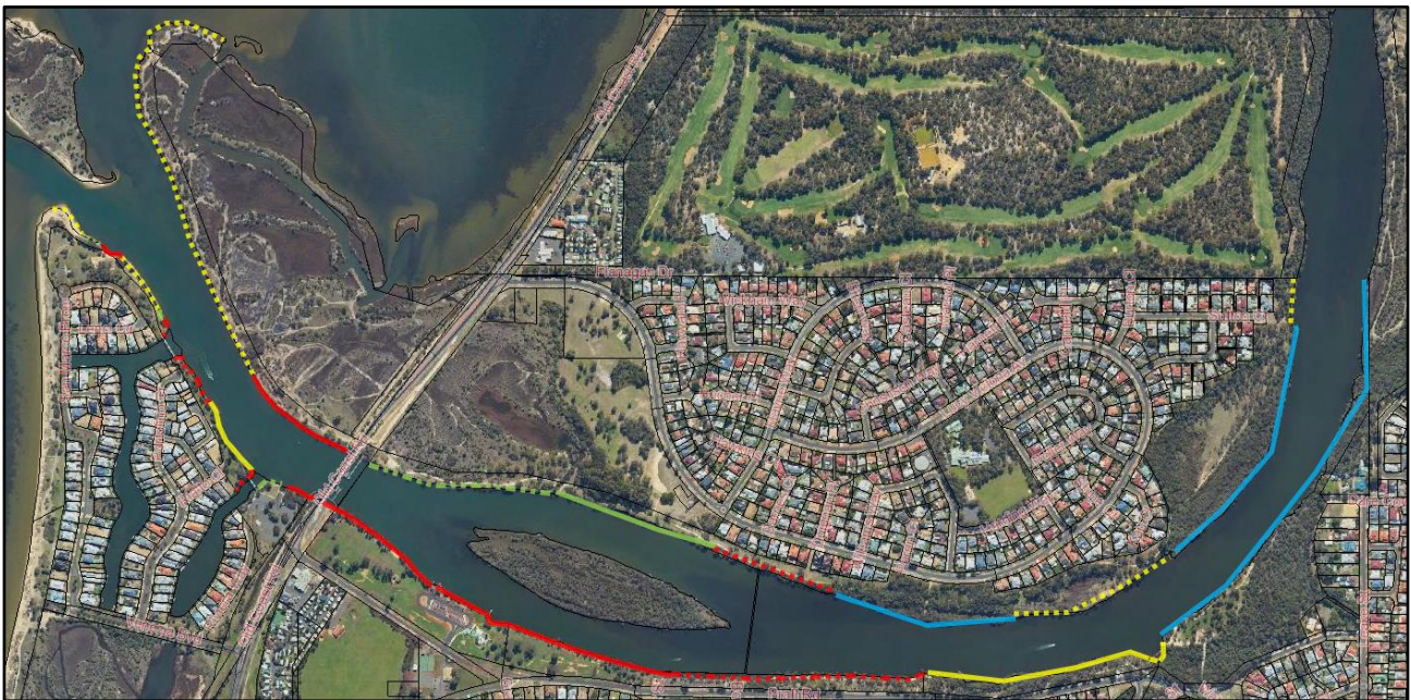
Figure 2-1 Priority of Foreshore Erosion Control (Image source: DWER 2018). Red = priority 1 (0-5 years), Yellow = priority 2 (5-10 years), Green = priority 3 (Greater than 10 years), Blue = no works required
