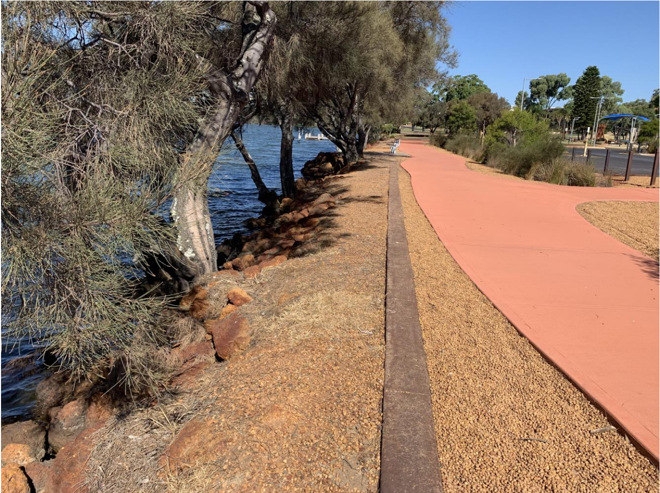
Figure 8-1 Eaton Foreshore – with Informal Rock Revetment, Narrow Strip of Vegetation and Dual Use Path in Close Proximity
