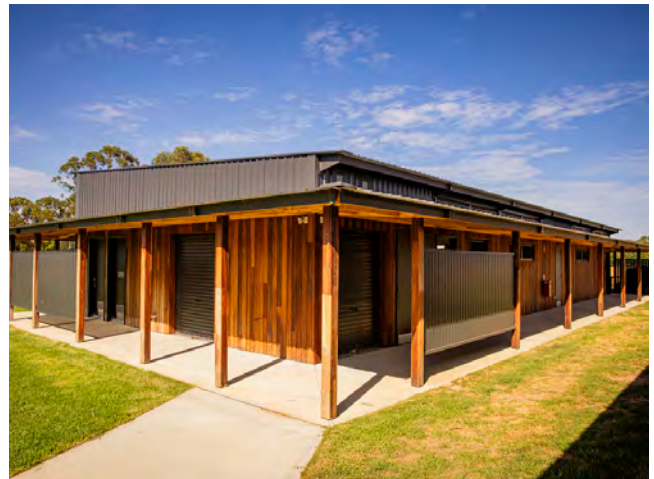
Project: Wells Recreation Park Redevelopment, 2021.
