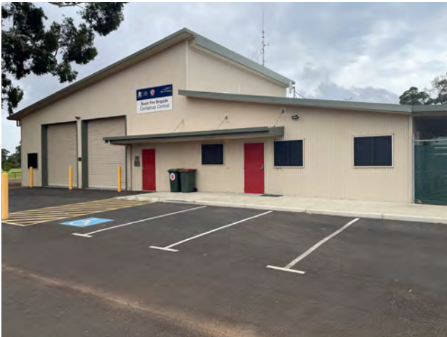
Project: Dardanup Centrais Volunteer Fire Brigade and Wells Change Rooms Building, 2022.
