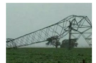
24-hour structural movement monitoring
