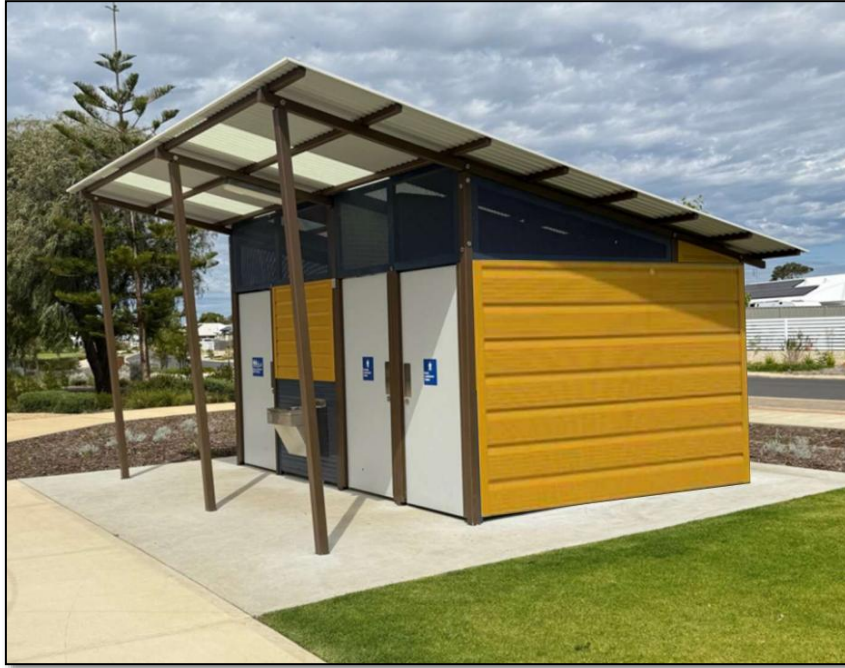
Image showing a public toilet with “Timber Look Aluminium Cladding”
