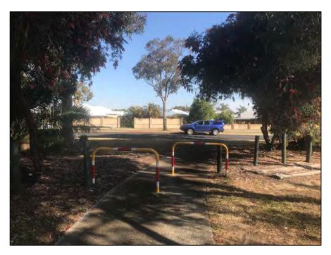
Finding 2.4 – Grab rails incorrectly installed and difficult to see at night.
