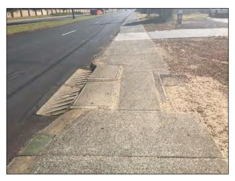
Finding 2.9 – High fall off the edge of the path at the side entry pits.
