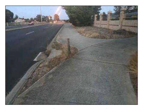
Finding 2.4 – Post on the edge of the path, very dangerous for cyclists in poor light conditions. Not conspicuous at all.
