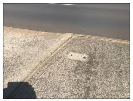
Finding 2.4 – Grab rails removed but holding down bolt still in the path, trip hazard. East of Hands Avenue.
