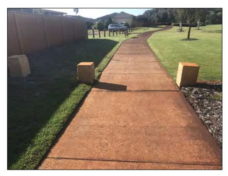
Finding 2.4 – Blocks on the edge of the path - should be 300 mm offset. Possible peddle snag for cyclists.
