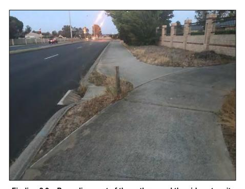
Finding 2.9 – Poor alignment of the path around the side entry pit.
