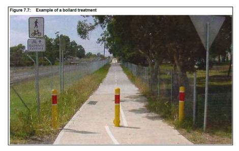
Finding 2.4 – Typical bollard treatment detailed in Austroads Guide to Road Design Part 6A: Paths for Walking and Cycling (2016).
