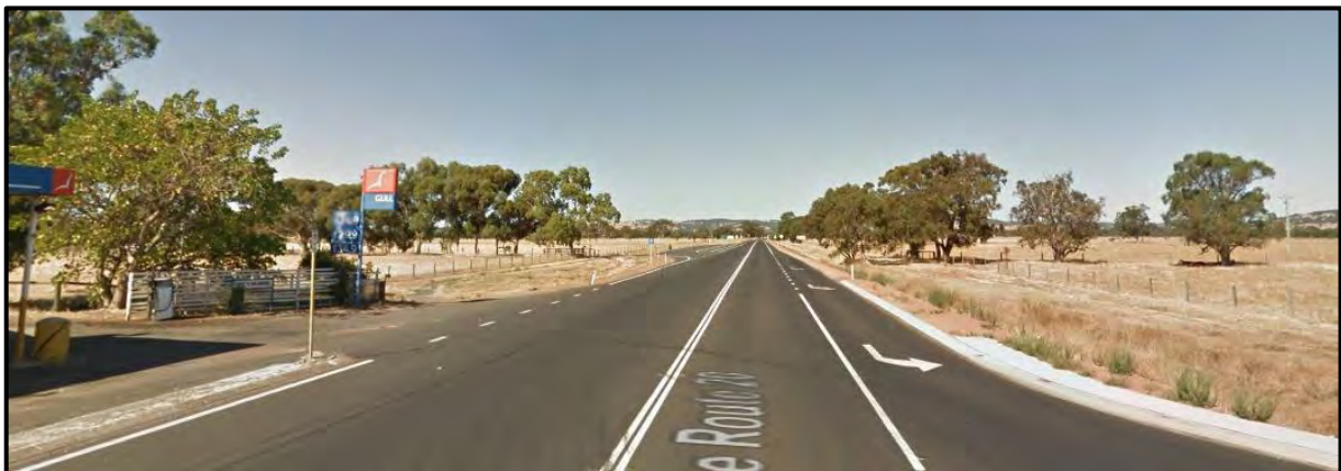
Figure 12 - Waterloo Road / South Western Highway Intersection Looking East
