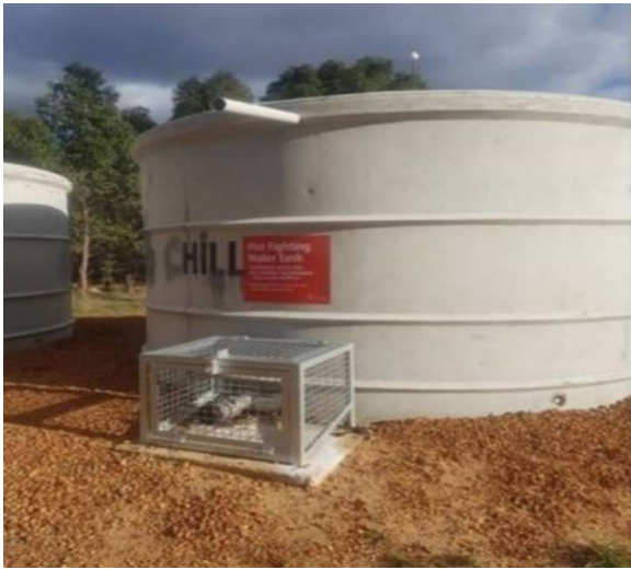
Strategic 47,000 Litre Concrete Tank & Protected Fittings
