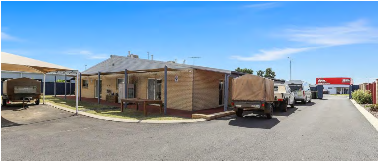
Photo 4: The rear of the existing building on the subject land.
