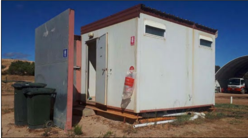
Existing amenities block
