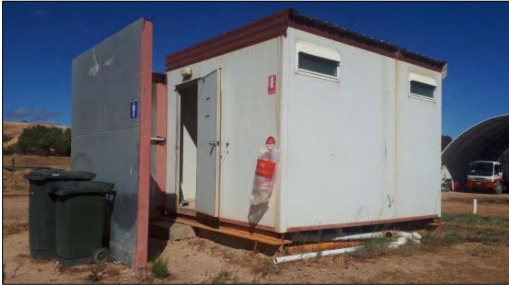
Existing amenities block
