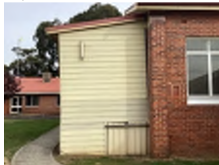
Showing examples of subfloor hatches
