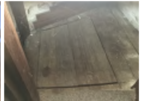
Showing examples of subfloor hatches found
