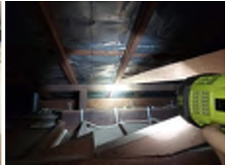
Showing example of insulation to the ceiling space
