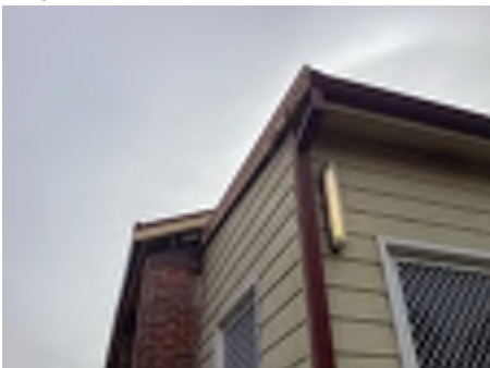
Showing no access to roof exterior due to height restrictions
