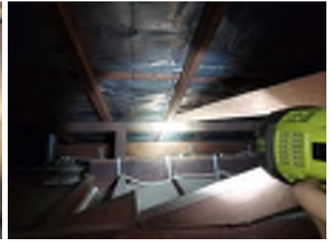
Showing example of framing and low clearance in the roof space
