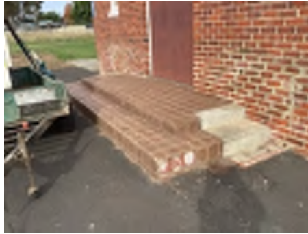
Showing examples of stairs
