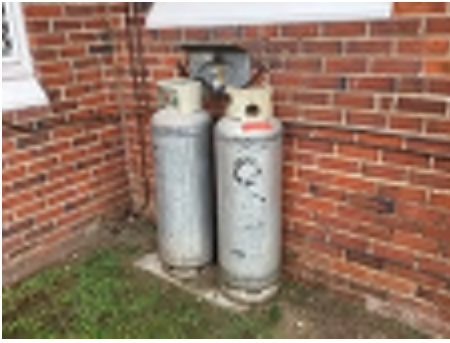
Showing gas bottle chain connection
