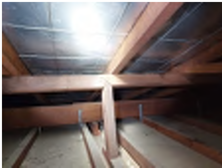
Showing example of insulation to the ceiling space
