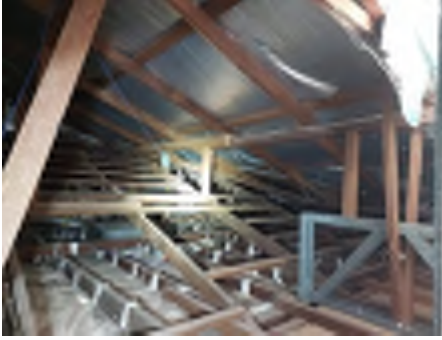
Showing example of framing and low clearance in the roof space
