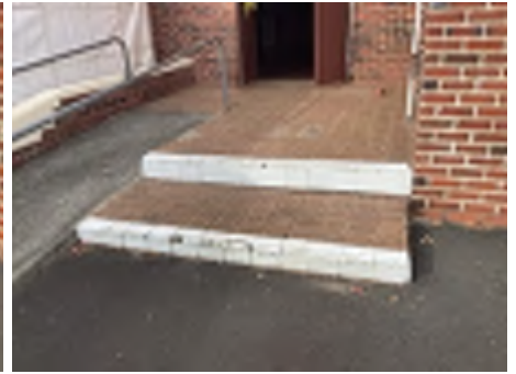
Showing examples of stairs
