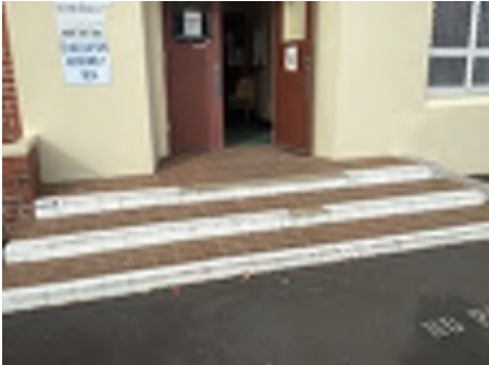
Showing examples of stairs
