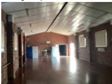
Showing example of wall, floor and ceiling coverings
