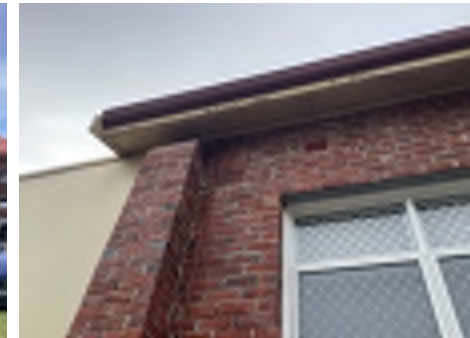
Showing no access to roof exterior due to height restrictions
