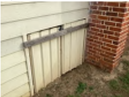
Showing examples of subfloor hatches
