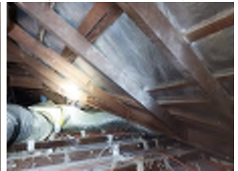
Showing example of framing and low clearance in the roof space
