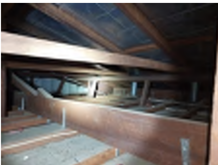
Showing examples of the roof space
