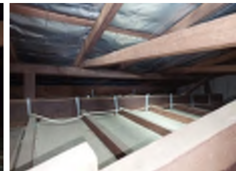
Showing examples of the roof space
