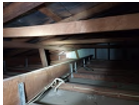
Showing examples of the roof space
