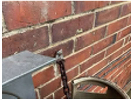
Showing gas bottle chain connection
