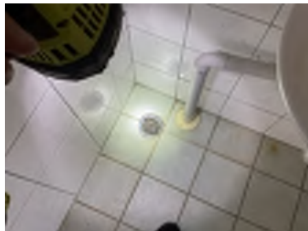
Showing examples of additional photos
