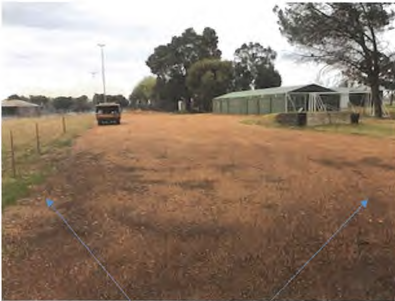
Figure 3 Parking Area too small in front of station
