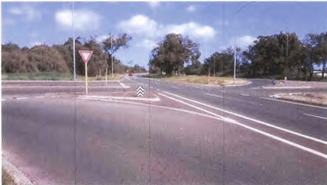
Photo 6: Seagull style intersection of Hynes Road with Forrest Highway.
