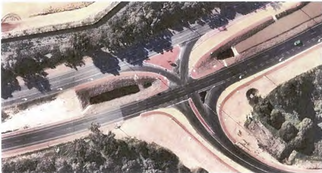
Figure 2.6: Upgrades under construction, August 2018
