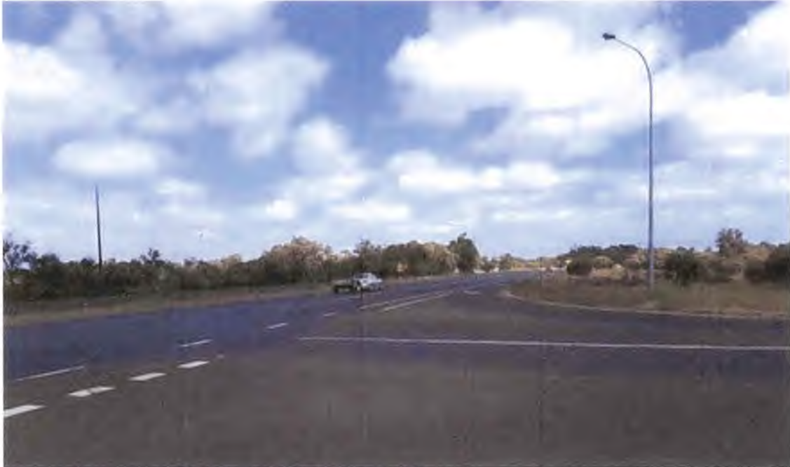
Photo 7: Intersection of Hynes Road with South Western Highway.
