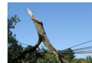
360° remote visual inspection
