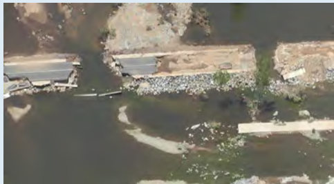
Hillside - Marble Bar Road (severe washout)
