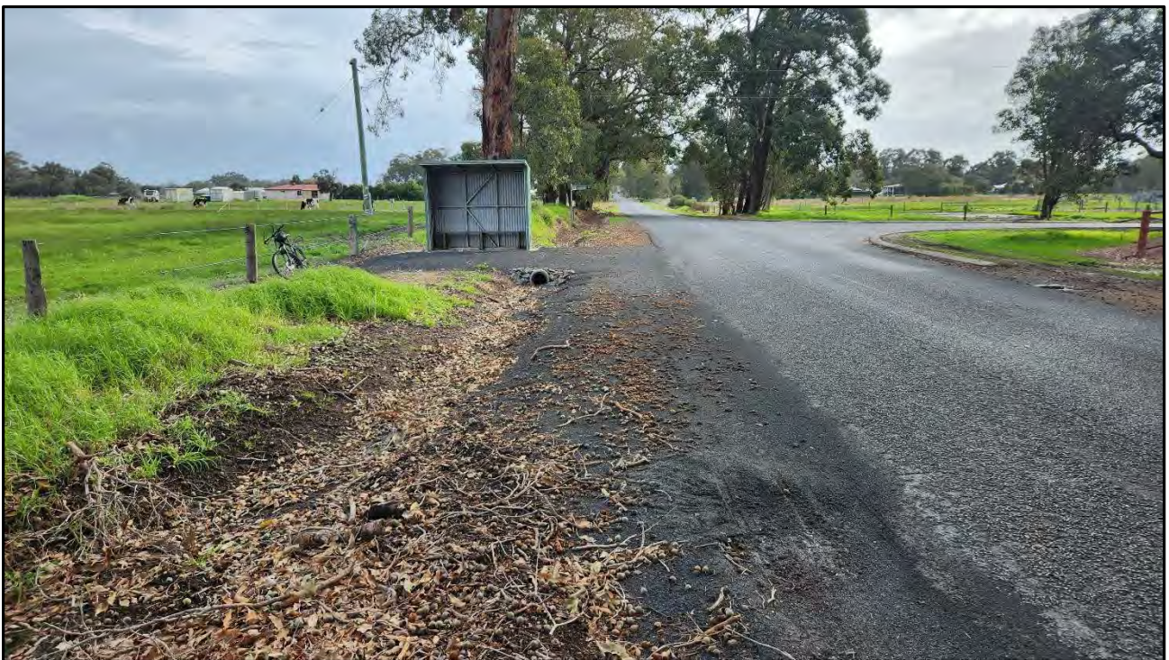
Photo 10: DN300 at northwest corner of site near Padbury Rd.
