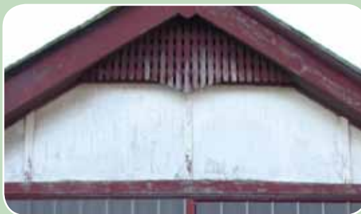
... and in the gable end of a garage
