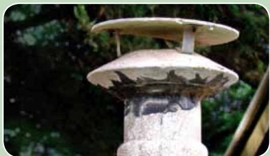
Asbestos cement flue and cowl
