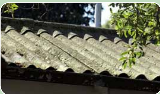
Asbestos cement corrugated roofing
